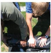
**Step 8**: Begin rolling from the furthest point away from the Port (Blower tube). (Doing so pushes air to escape as you roll.) Roll as tightly as possible. Keep the roll lined up, tuck any in extra material, and do not allow any part of the roll to sag. Slack rolls are difficult to move. Take your time and roll it tight.
