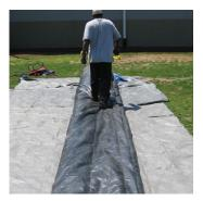
**Step 6**: Walk air out of the Inflatable by walking on the Inflatable towards the Port (Blower tube). (Doing so pushes air and allows air to escape.)
