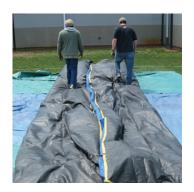
**Step 5**: Tuck in any extra material. (Leave Ports out to allow air to escape as you roll.)
